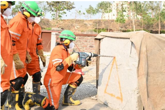
Collapse Structure Search & Rescue (CSSR)
